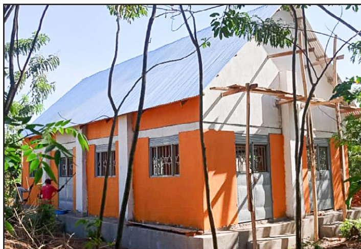
The finishing touches were applied to the new synagogue.
