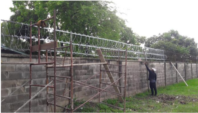
Repairing the wall in the Ashkenazi Cemetery
