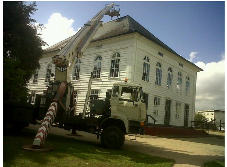
Roof repair - another challenge overcome!
