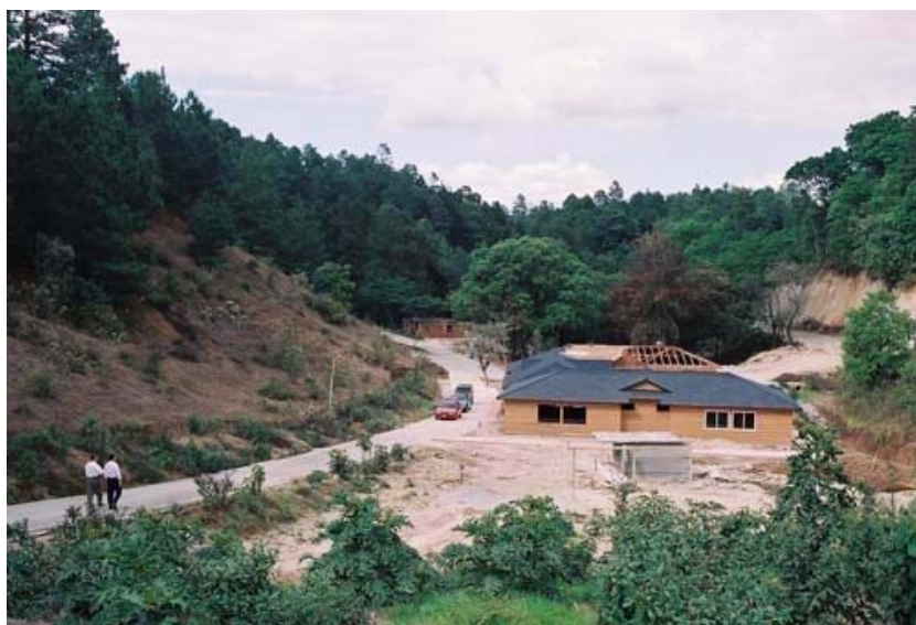
Construction at Har Carmel, Guatemala
